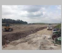
The wet soils were then imported via 8 wheel tippers and lime was added using Pryor Stabilisation's Terragator Spreader and Fendt 939 with mixing drum.
